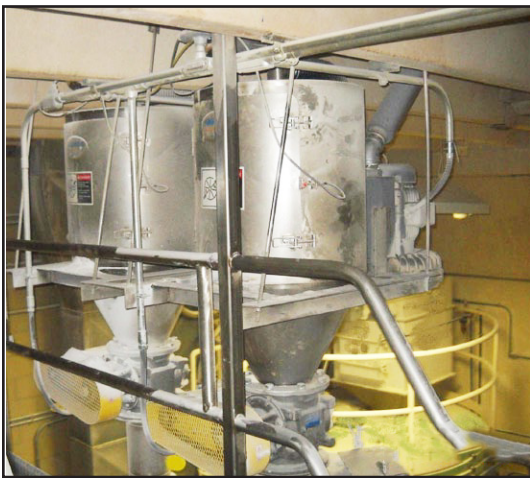
The pneumatic vacuum conveyors move the bulk powder about 150 ft (45.7 m) 8 hours a day, 5 days per week.
