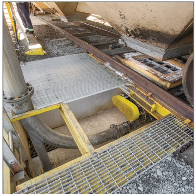
18” rotary feeder control feeds the prill into the Tubular Drag Conveyor.
