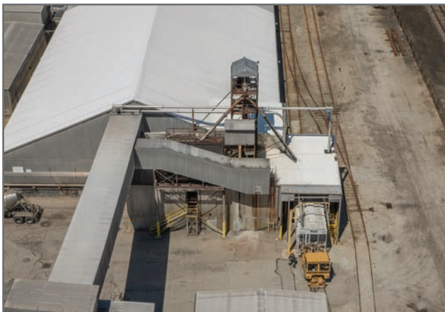
Overview of Tubular Drag Conveyor: Elevates up from the railcar house (right side photo), and then moves material to discharge point at the belt conveyor tunnel (left side photo).
