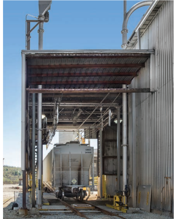
Carry and return sides of conveyor on either side of pit.
