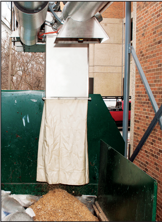
Soiled bedding is removed via the system's tubular drag conveyor and empties into an outside dumpster, eliminating the need for lab assistants to lift heavy bags into dumpsters, or additional contact with contaminated bedding.
