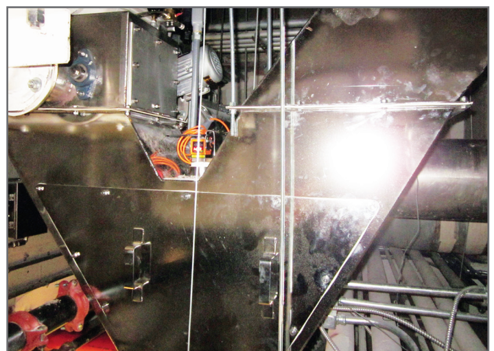
The custom engineered Wye piping configuration was designed to connect the 3rd floor stand pipe where the 1st and 2nd floor Tubular Drag conveyors feed the main conveyor.
