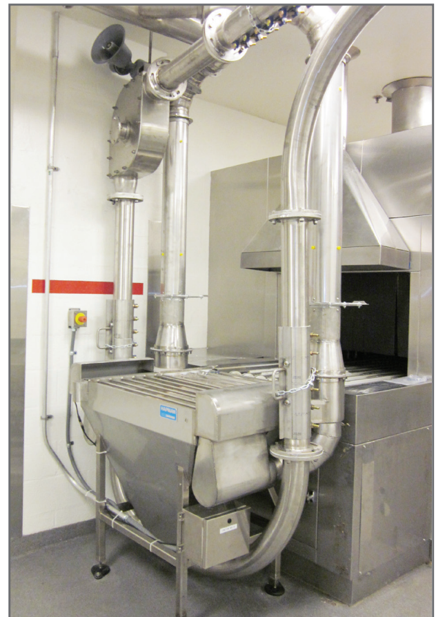
Based on technician feedback from using a cardboard model, the cage dump station with an integral HEPA air filtration system, was mounted directly in front of the tunnel washer, and significantly streamlined the process.
