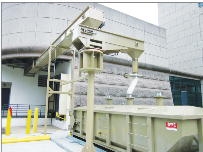
Located just outside the facility, the 45-foot conveyor unloads the briquettes into a custom designed container, featuring an automated load-out arm.
