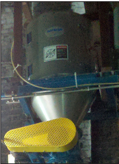
Hapman Model 24 Vacuum Conveyor installed at the Werner G. Smith facility.
